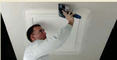
4. Tape and apply drywall compound.
