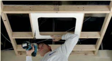
2. Mount Stylemark surround with drywall screws.
